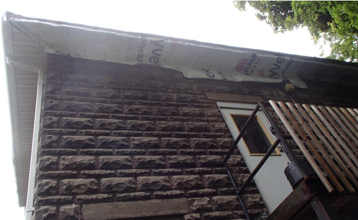
Photo: Soffits now have Tyvek covering eaves on south side - concern this is obstructing the air flow in the attic.
