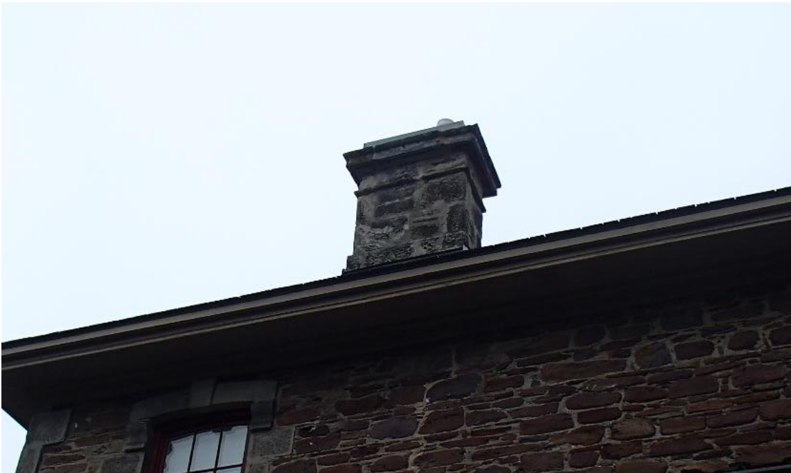
Photo: The chimney work is complete
