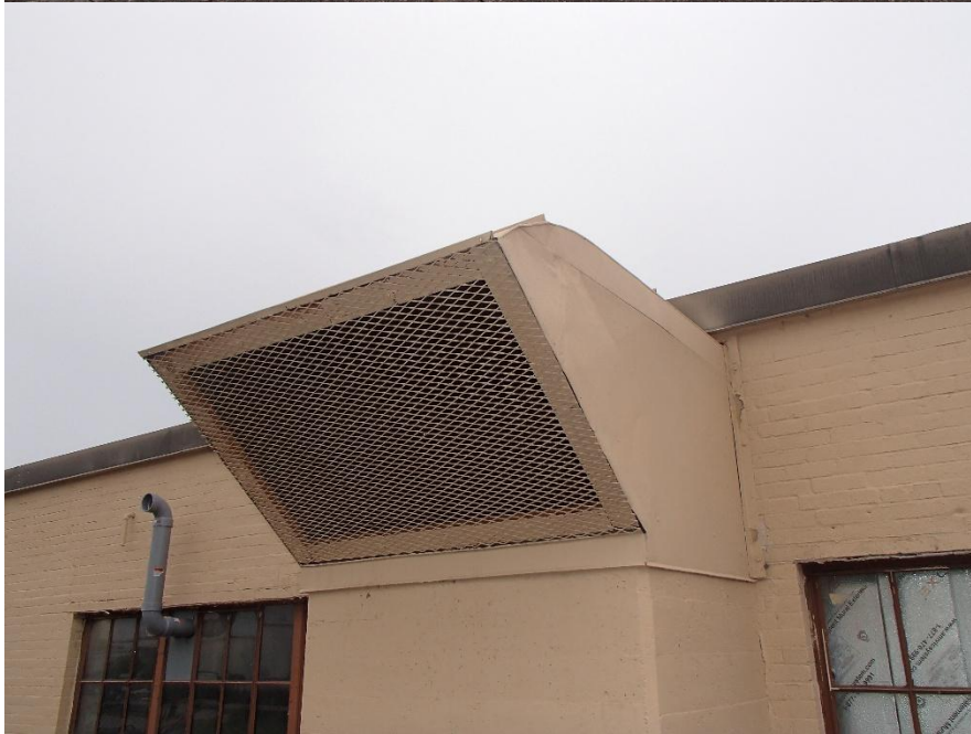
Vent repaired on east side and grill installed.
