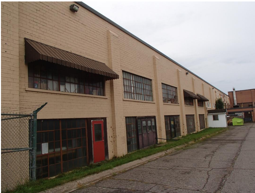
Photo: West wall painted and window pane replacement.
