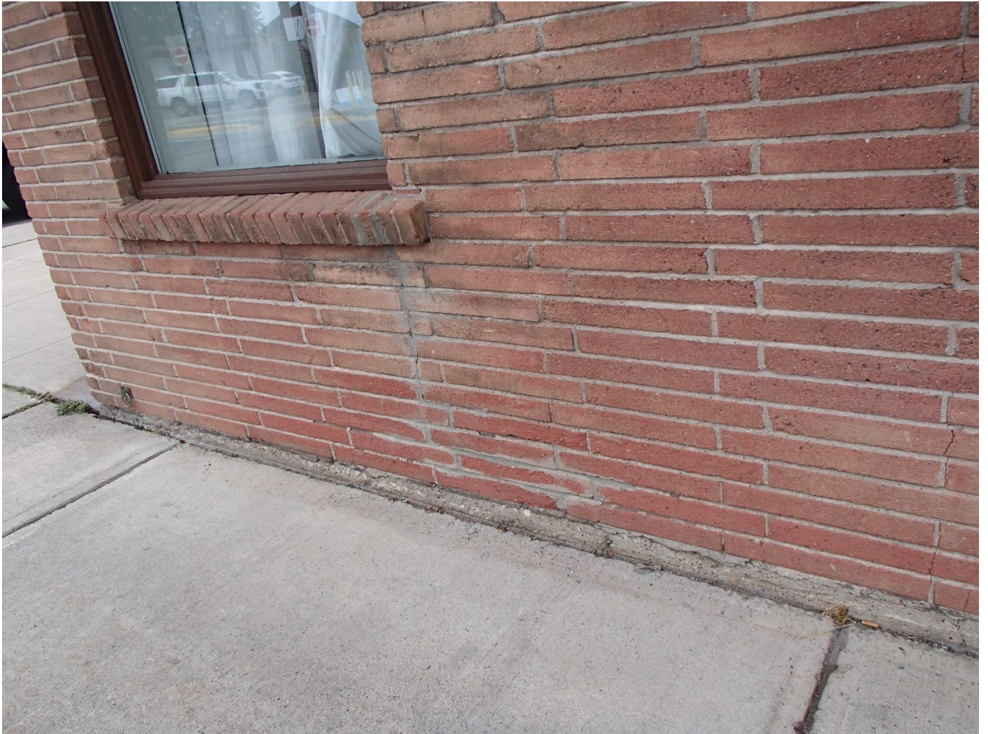
Photo: West wall – brick repair has been completed
