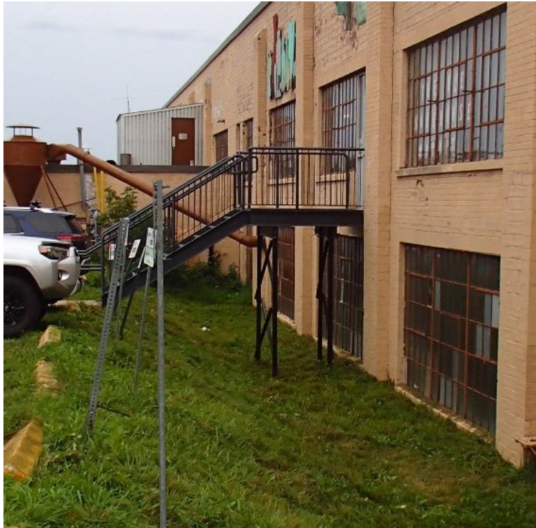
Photo: New staircase on east wall
