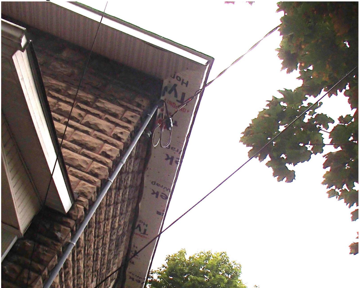
Photo: Soffits now have Tyvek covering eaves on south side - concern this is obstructing the air flow in the attic.
