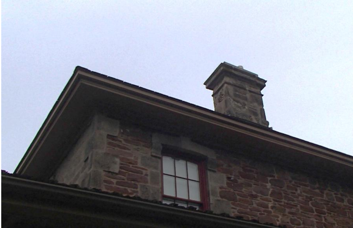
Photo: Stonework completed on the chimney at 10 Kensington Terrace.
