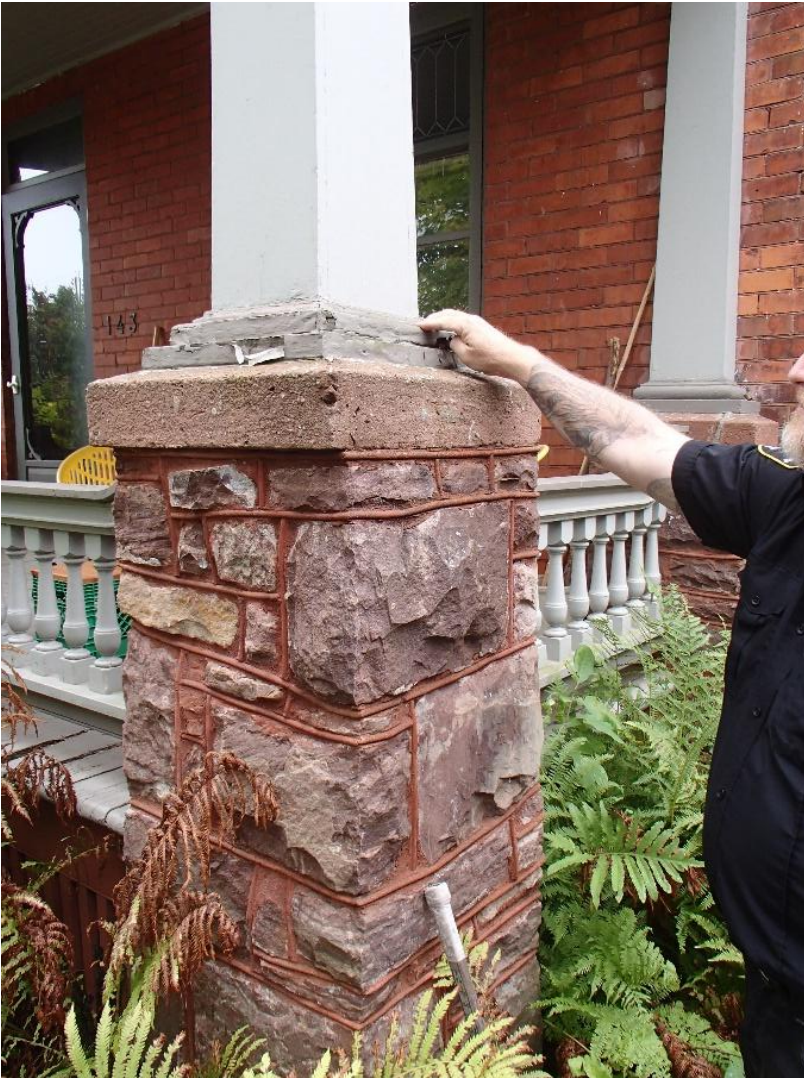
Photo: Porch Column
