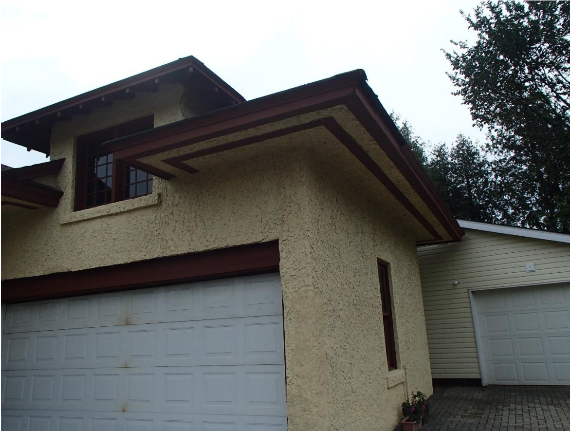
Photo: Front of house garage
