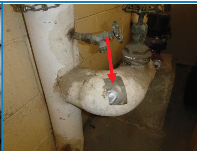
Photo 6: View of the asbestos containing paring cement insulation (see arrow) observed to be taped and in fair condition on water meter within Receiving area of the subject building.
