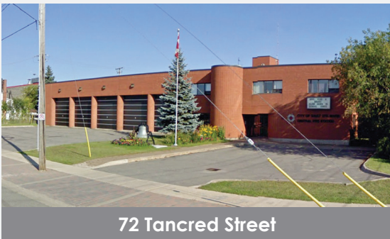
Main Fire Hall, Station 1
