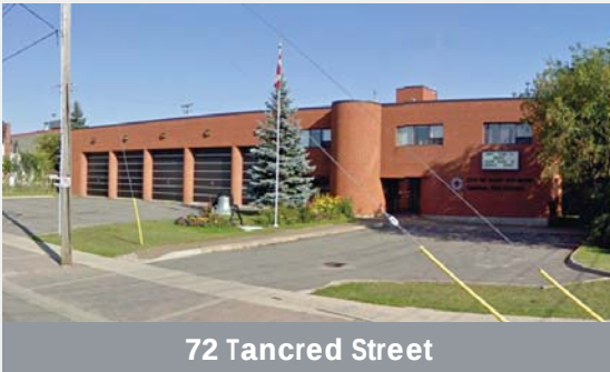
Main Fire Hall, Station 1
