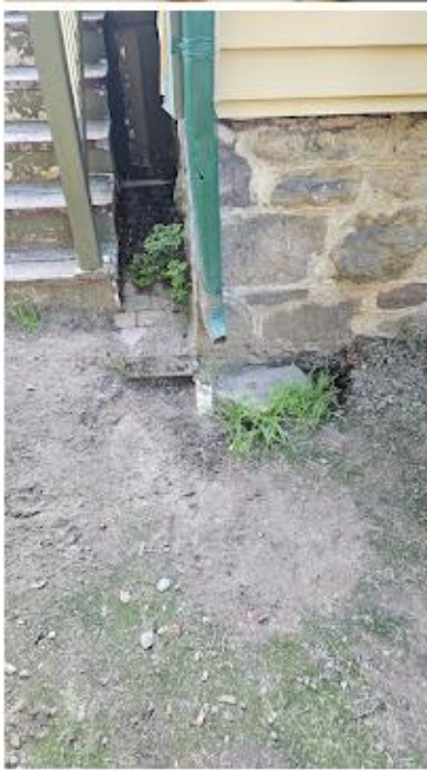
Photo: Foundation repair
