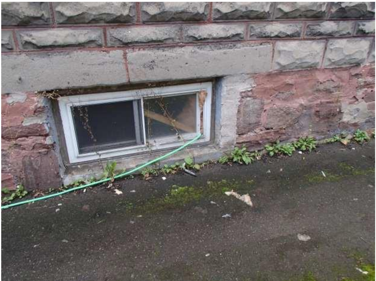
Basement window – more insulation sticking out
