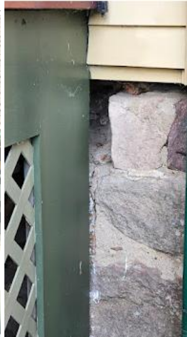
Photo: Foundation Repair
