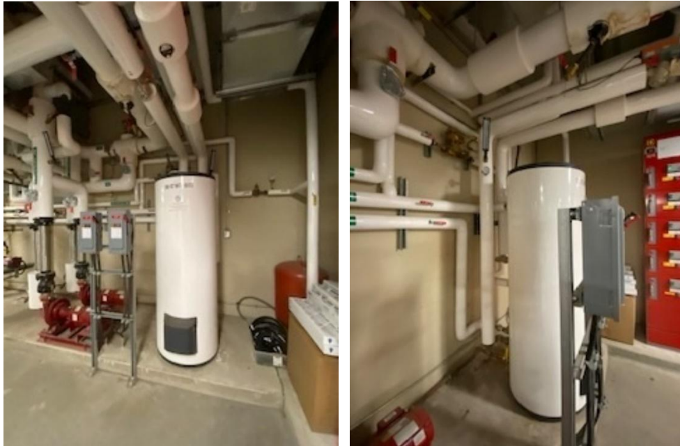
Figure 16. DHW Tank
