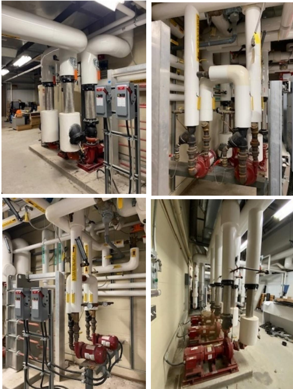
Figure 15. HW Circulation Pumps
