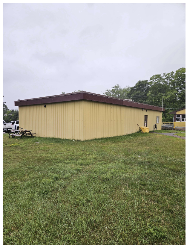
Photo No. 2 - Administration Building (Northeast)
