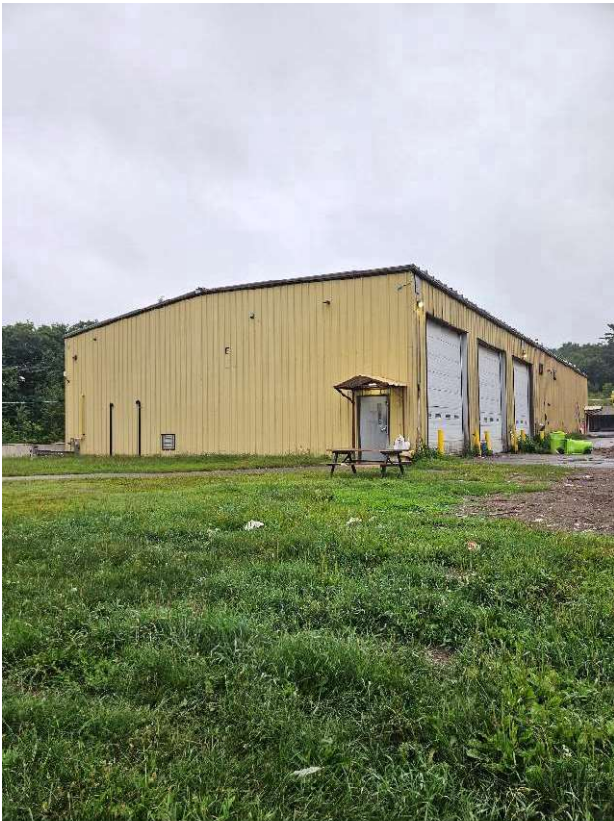
Photo No. 3 – Maintenance Garage (Southeast)
