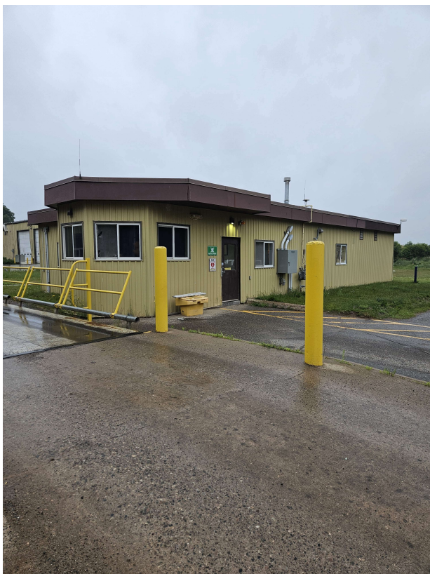
Photo No. 1 - Administration Building (Southwest)
