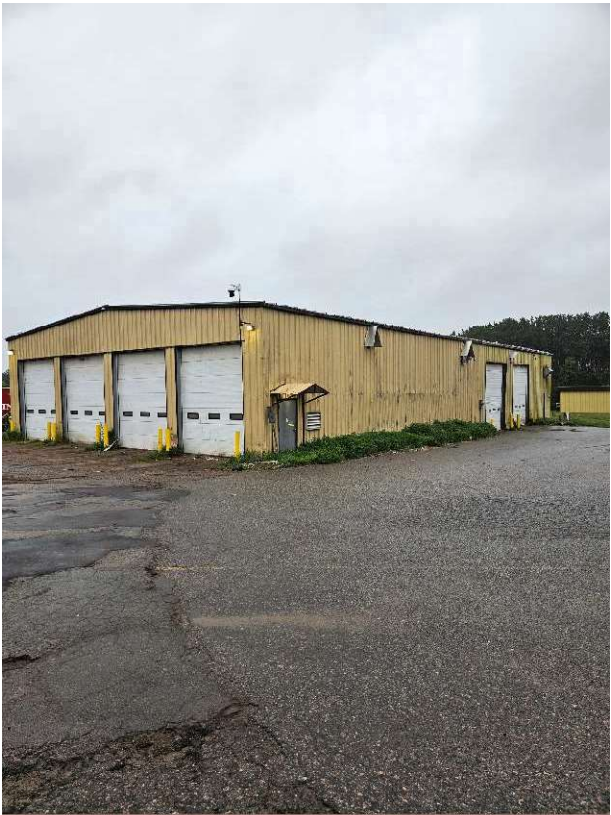
Photo No. 4 – Maintenance Garage (Northwest)
