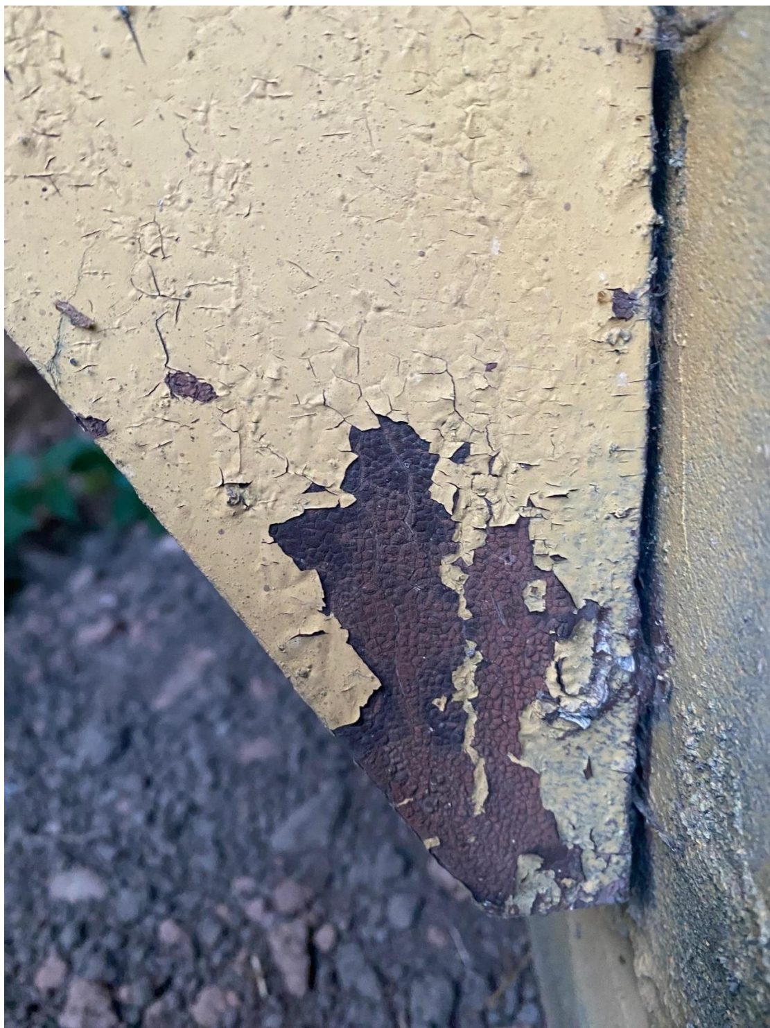
Photo: Brown paint on the trim underneath the current yellow paint.
