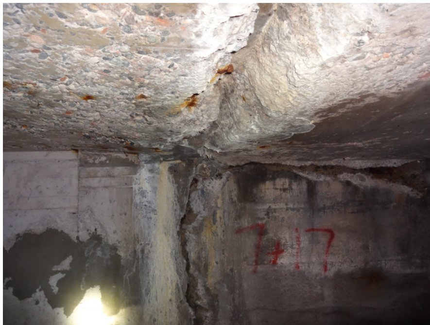
Deteriorating joint just north of St Andrews Terrace –photo by STEM Engineering
