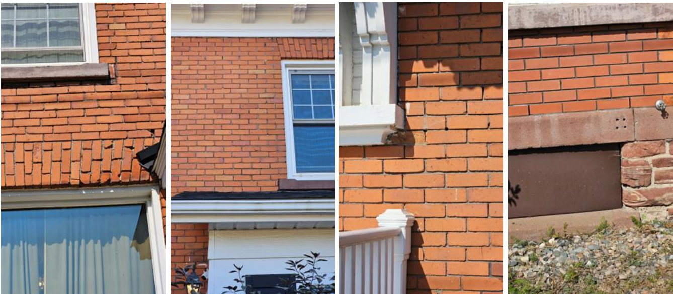
Photo: Spalling brick
