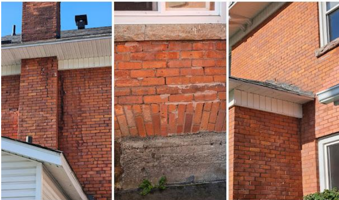
Photo: Spalling brick work
