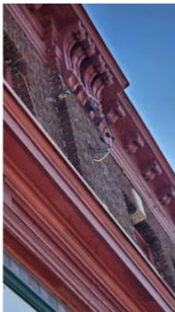
Photo: Loose wires
