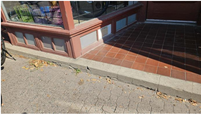
Photo: Cracked concrete
