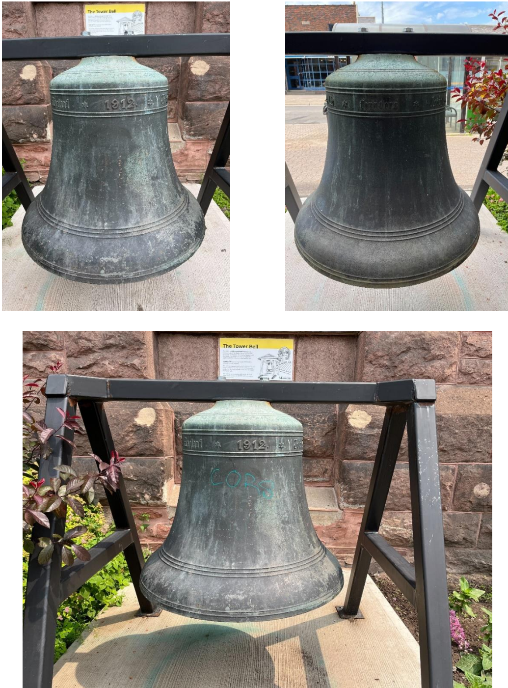
Figure 4: Before conservation process - photos above from front and rear view of the bell before the second vandalism event and the photo below of the front side of the bell after the second vandalism (photo by the writer, summer 2023)
