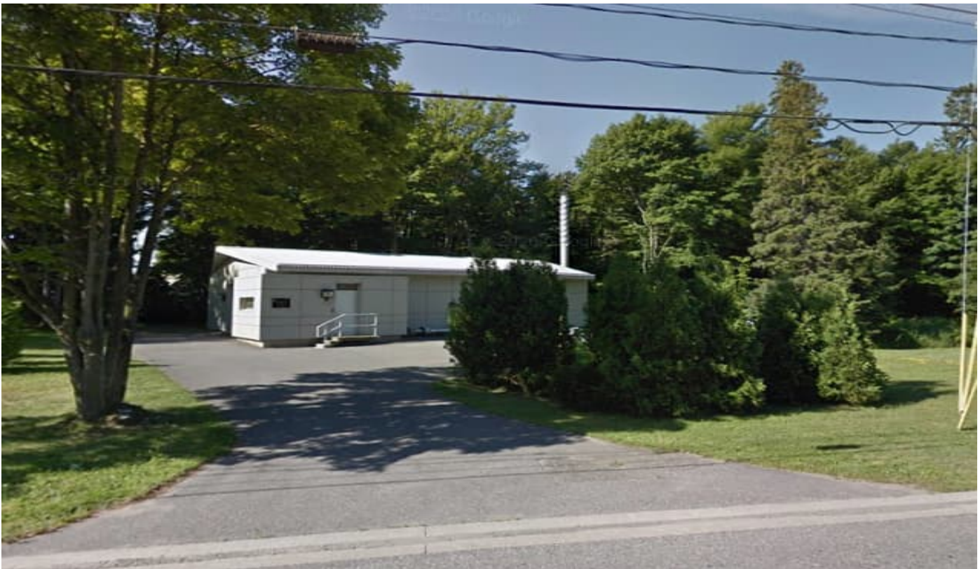
Clark Creek Lift Station
