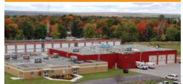
Station 4 - Regional Emergency Response Centre (RESC)
