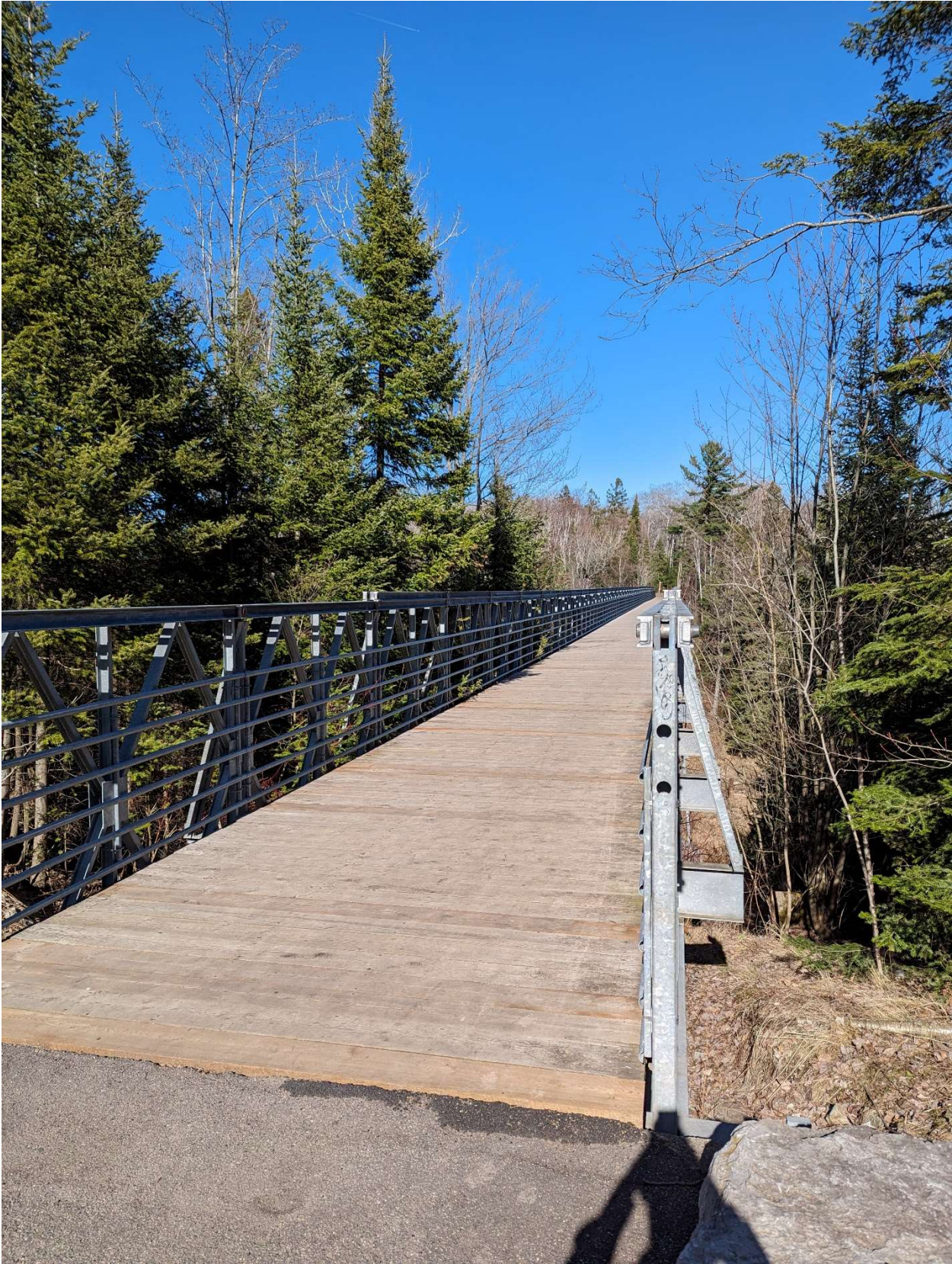
Fort Creek Bridge – Near Third Line East
