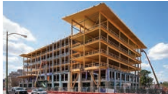
Mass Timber Construction
