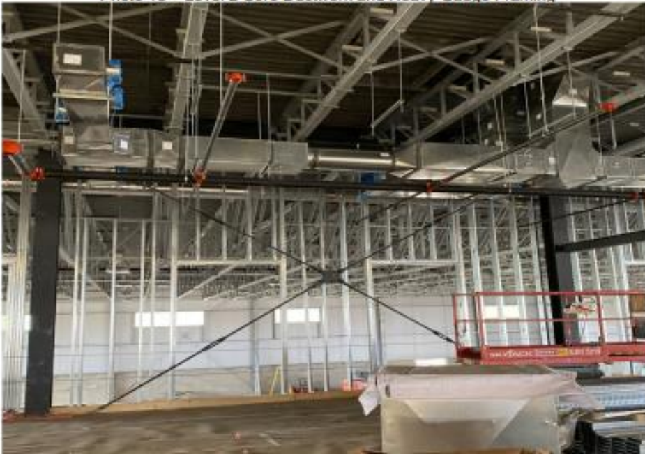
Photo 13 – Level 2 Core Ductwork and Heavy Gauge Framing
