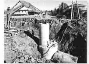
Pim Street Storm Sewer Upgrades
