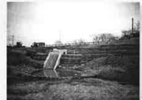
Gladstone Ave. Stormwater Management Pond Control Structure
