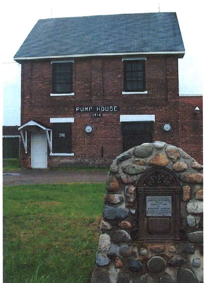
Steelton Pump House established 1914.
