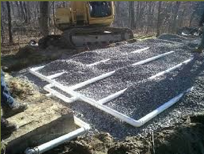
A typical class 4 septic system under construction
