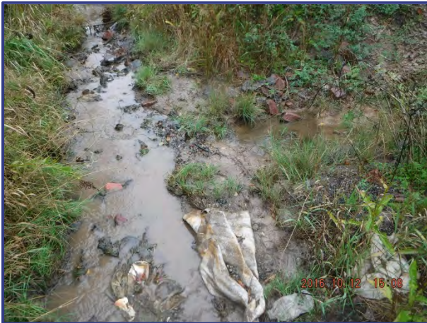
Photograph 21: Sediment of constructed drain at center of Sackville Site.
