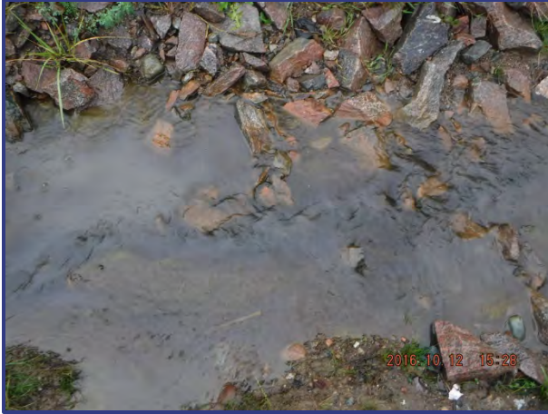
Photograph 19: Sediment of constructed drain at south edge of Sackville Site.
