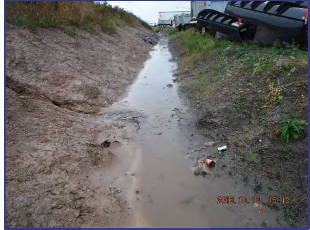
Photograph 20: Constructed drain at center of Sackville Site.
