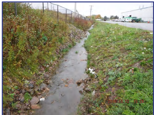
Photograph 186: Constructed drain at south edge of Sackville Site.
