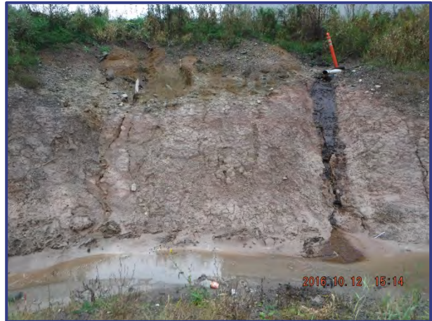
Photograph 22: Banks of constructed drain at center of Sackville Site.
