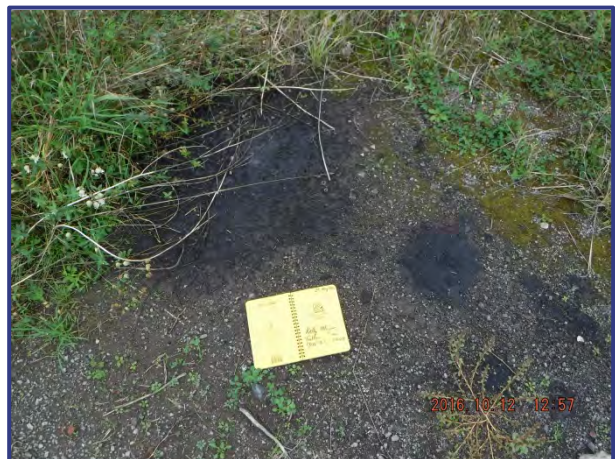
Photograph 6: Stains suggest soil contamination by automotive fluids at Huron Site.
