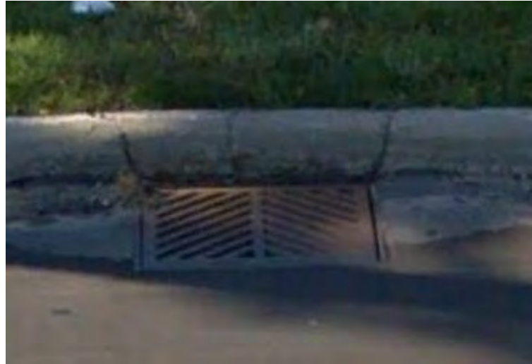
Figure 7: Drainage Grate on Northern Avenue 13
