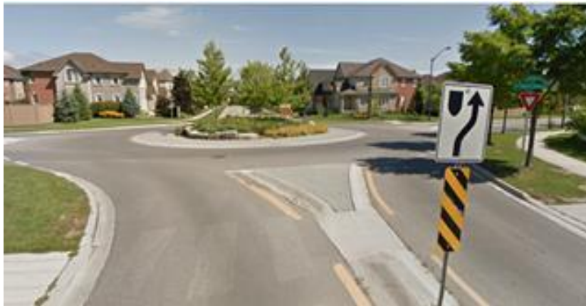
Figure 8: Small-radius Modern Roundabout
