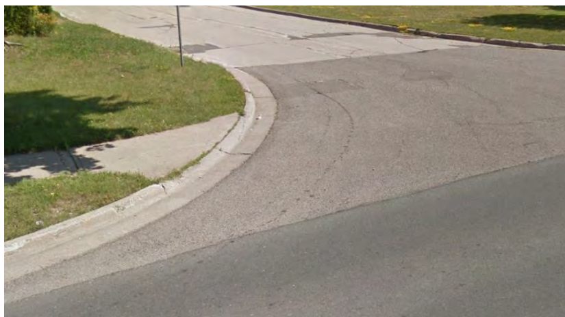
Figure 5: Depressed Curb on Northern Avenue at Anita Boulevard 10
