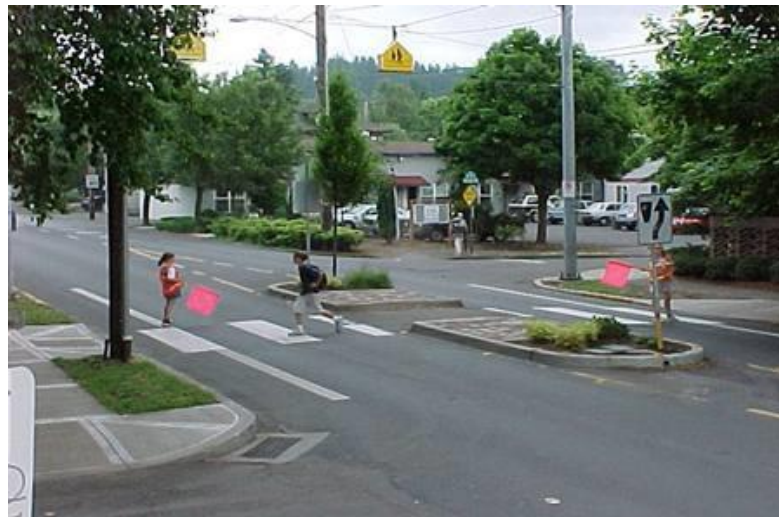
Figure 14: Raised Median Island
