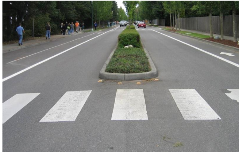
Figure 13: Raised Median Island
