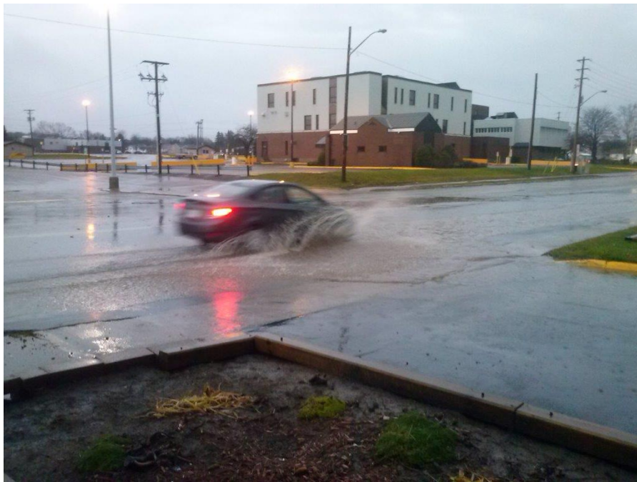
Ponding in road sag in front of 205 McNabb Street Nov 17/13
