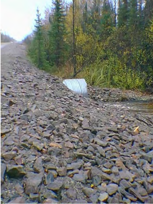
An example of a properly stabilized bank using rip-rap can be seen at Mile 10 on the Blueberry Road northeast of Longlac.
