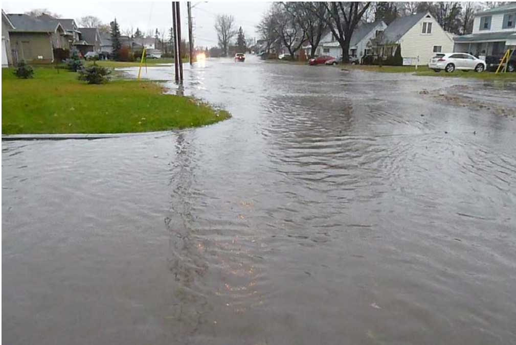
Surface Flooding at road sag point - MacDonald Avenue at Brien Avenue Nov 17, 2013
