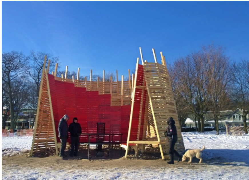
Figure 4-7: Example of warming station, design and image by Susan Drysdale for the Toronto Beaches Winter Stations Design Competition
