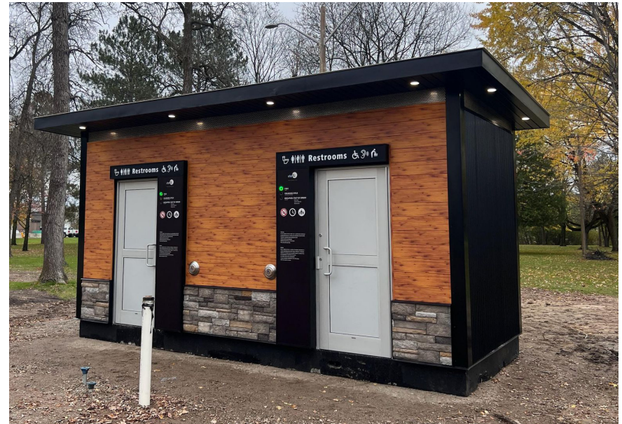
Figure 4-8: Urban Blu self-cleaning washroom in Fort Francis, ON
