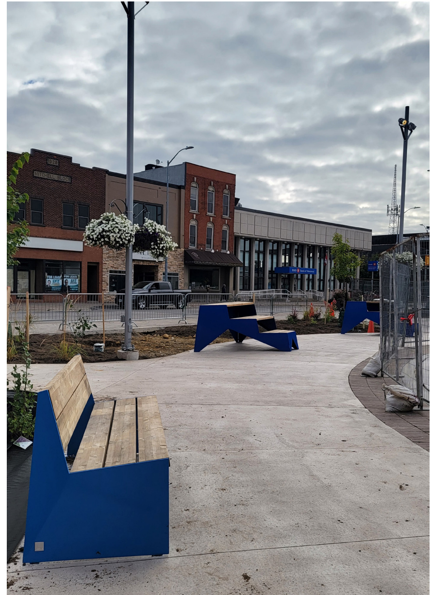
Figure 1-5: Work underway for the new Downtown Plaza, Fall 2023
