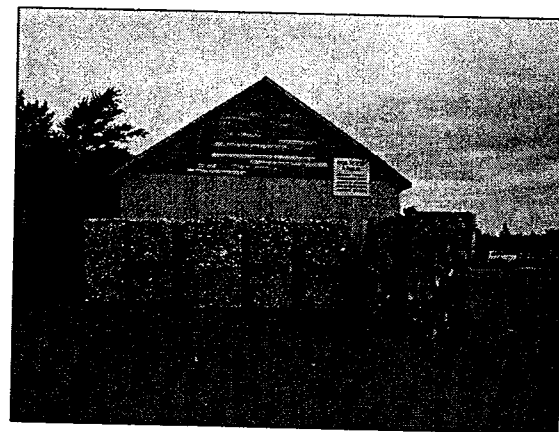
Photo No. 3 - South Side of Storage Building
