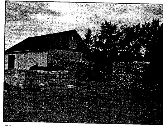
Photo No. 1 - Northeast Corner of Storage Building
