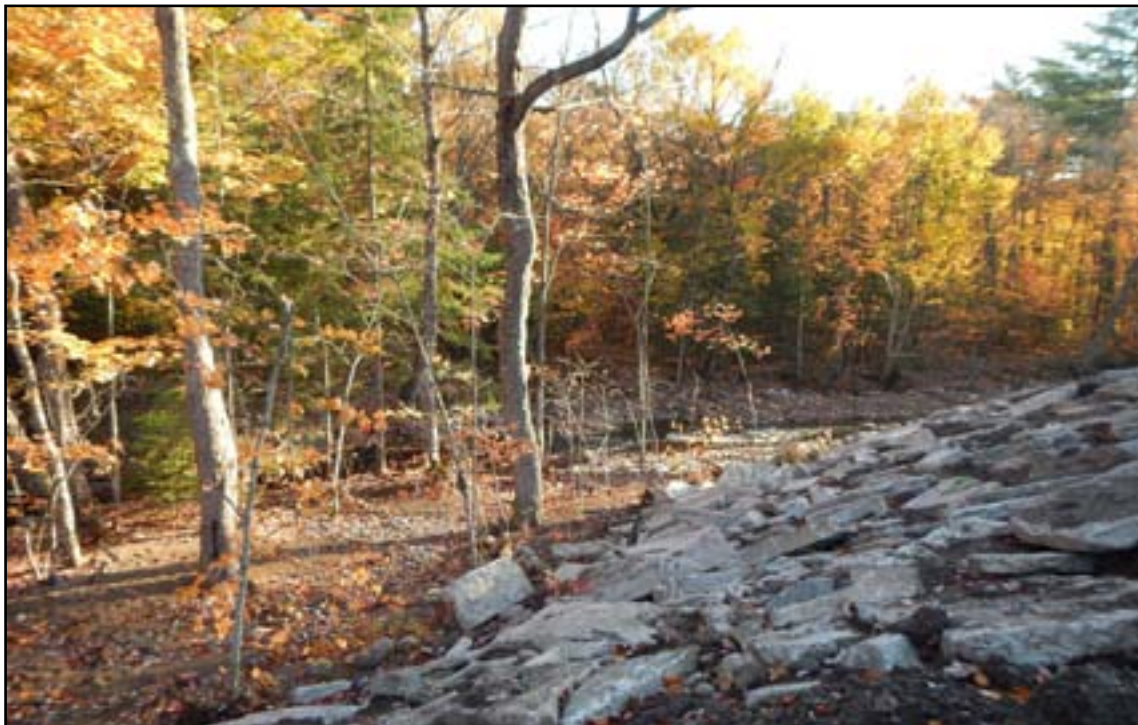
Photo 2. Canon Creek and erosion remediation, Area D.
