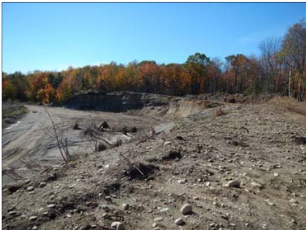
Photo 46. Earthmoving activities, Area E1.
