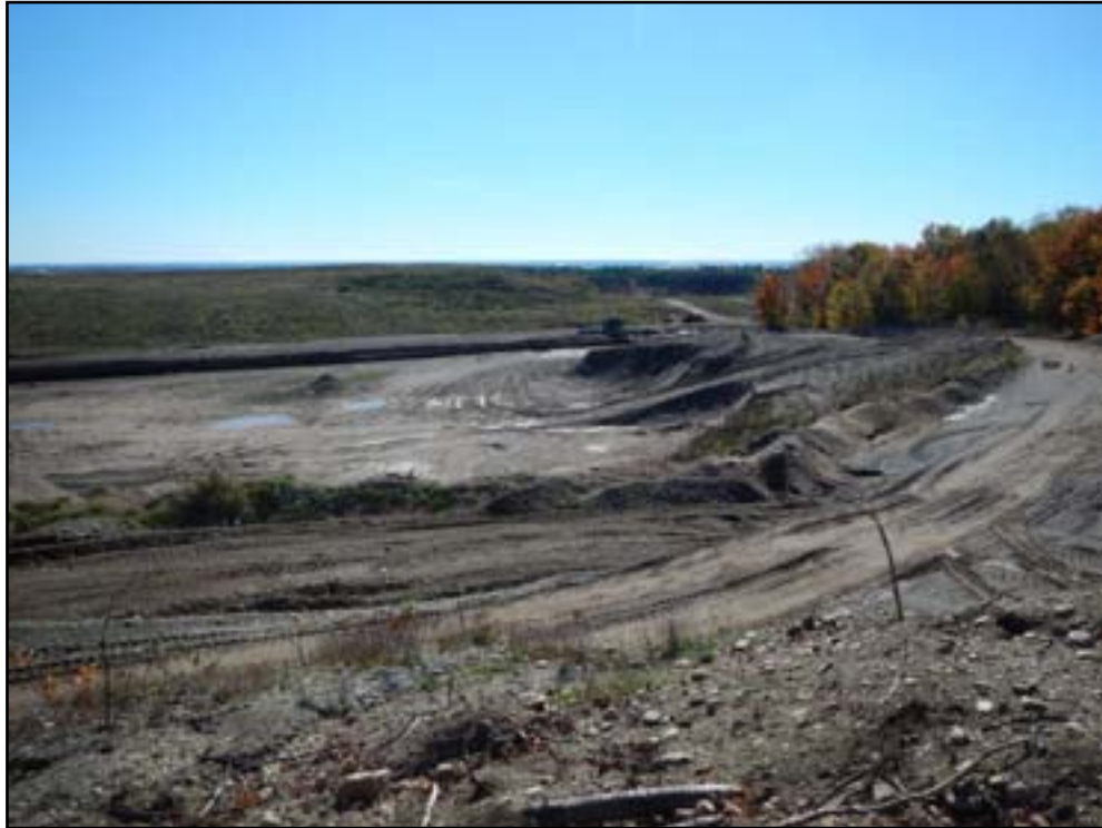
Photo 47. Earthmoving activities, Area E1.
