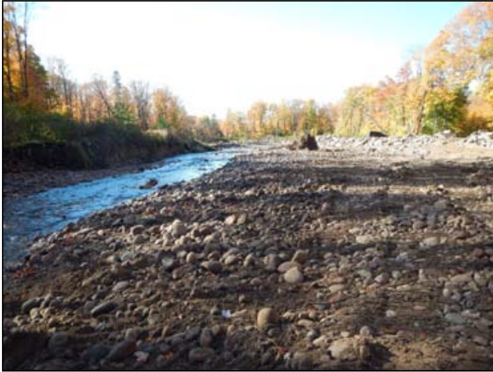
Photo 69. General view of the erosion at Canon Creek, eastern side of subject property.
