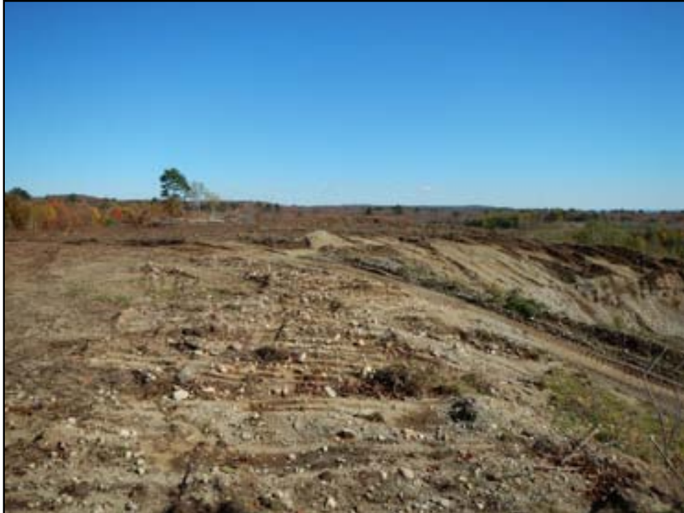
Photo 48. Earthmoving activities, Area E1.
