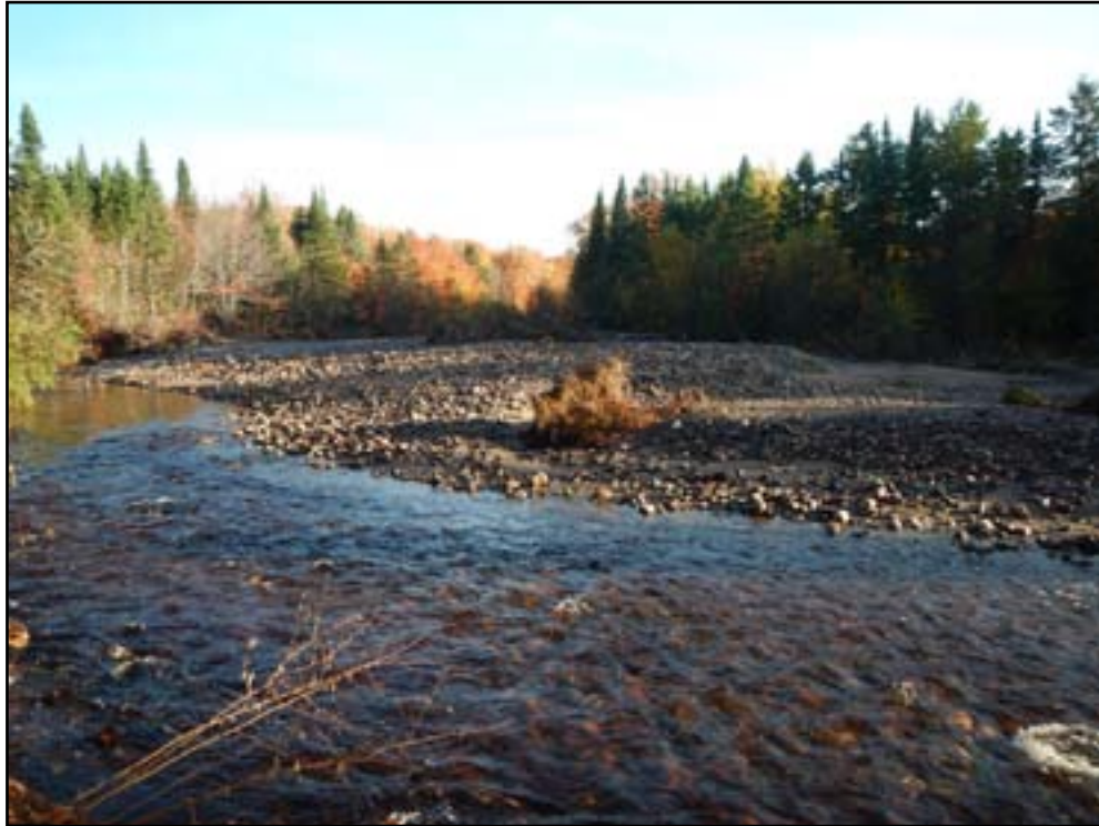
Photo 61. Canon Creek, erosion.
