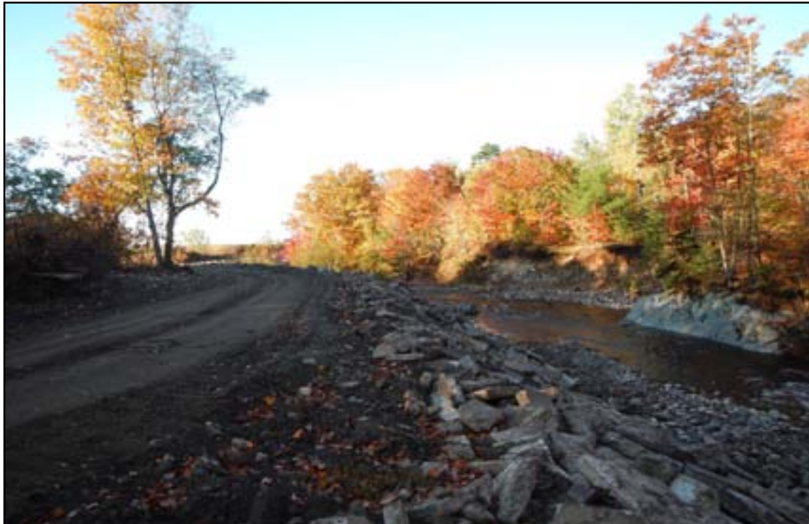
Photo 1. Canon Creek, and erosion remediation, Area D
