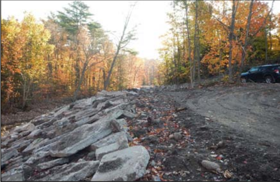
Photo 3. Canon Creek and erosion remediation, Area D.
