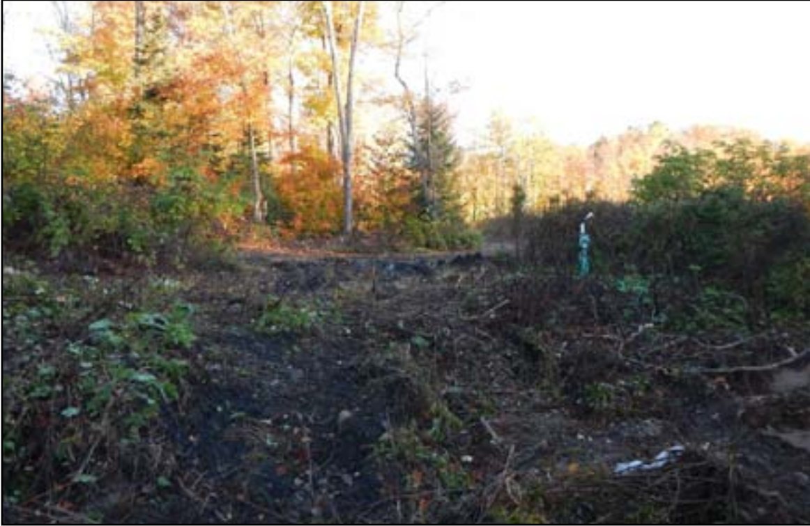
Photo 55. Erosion at Canon Creek, Area I.
