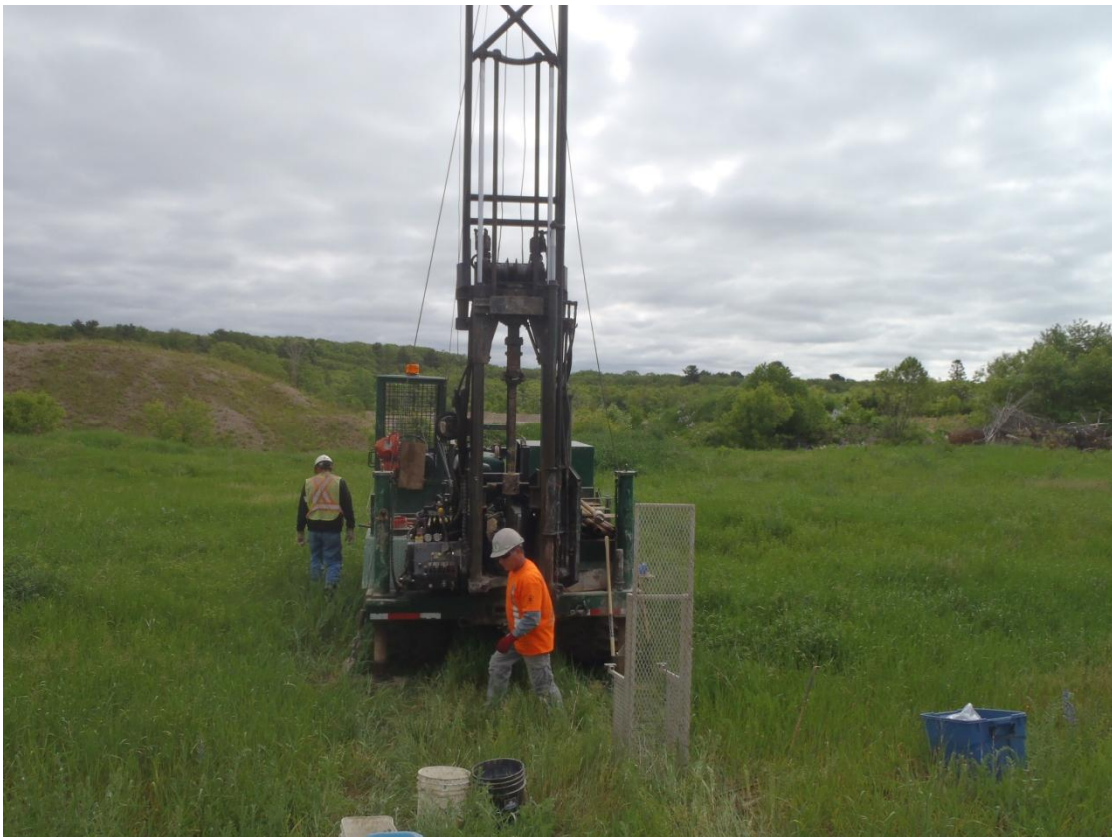
Photo 02: General site view, TH13-01, looking northeast
